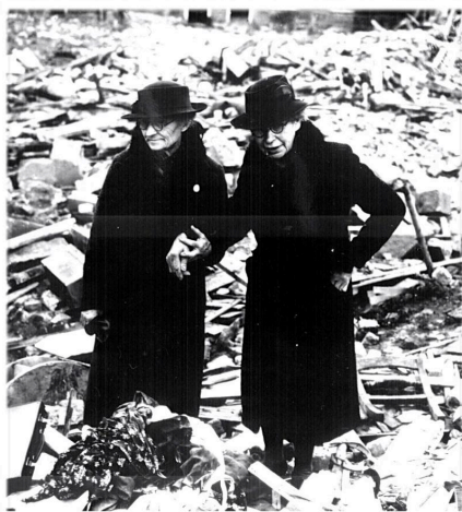
Two bewildered ladies stand amid the ruins of St. Bartholomew's almshouses, Newbury, destroyed by the same bomber which struck St. John's Church
